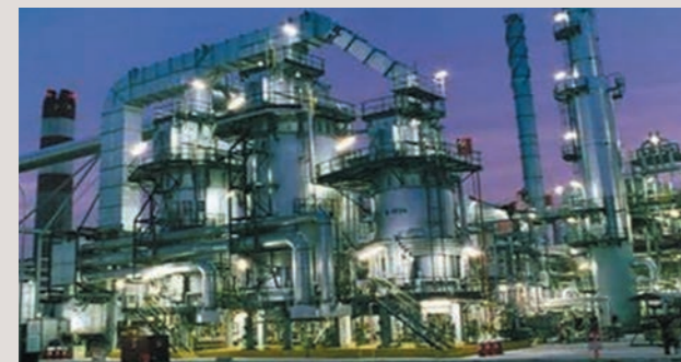
IOCL Panipat Refinery
