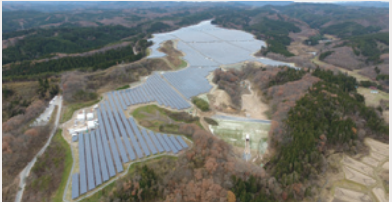
Furukawa Mega Solar Plant
