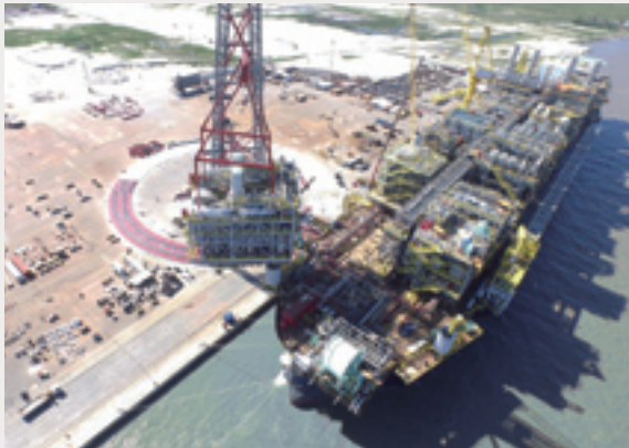
Modules onto the hull
