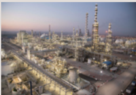
Ethylene and polyethylene plant
