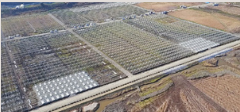
Frame mounts installed at the construction site
