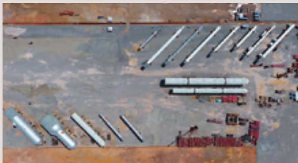
Top: Ultra-tall towers being unloaded at the construction site
