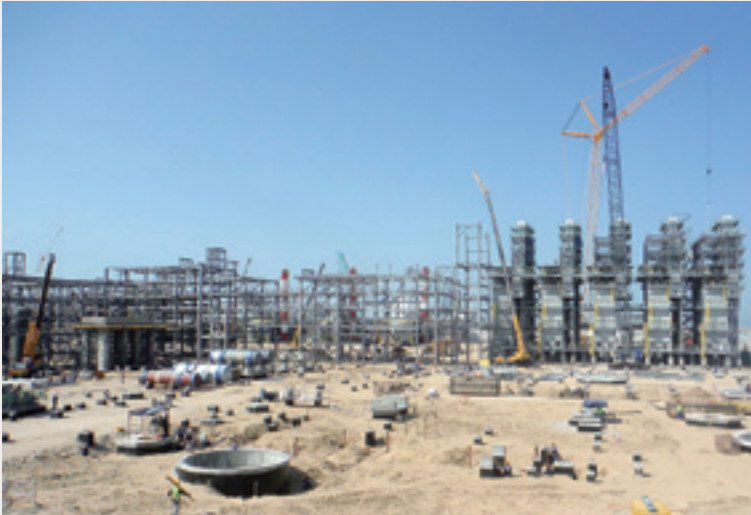
Construction commences on the ethane cracker
