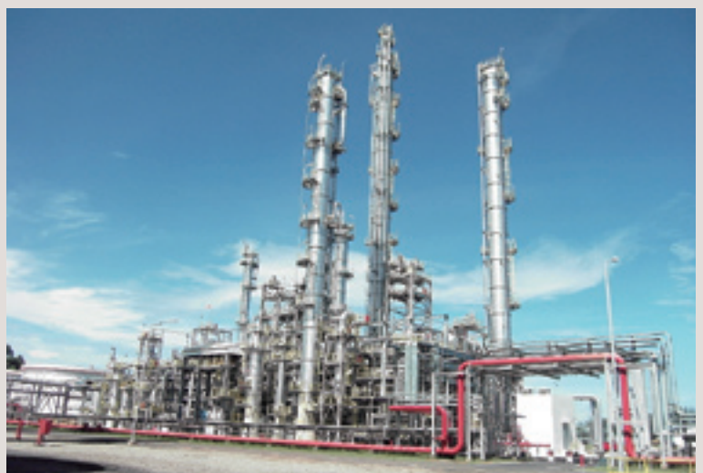
Butadiene plant completed in 2013
