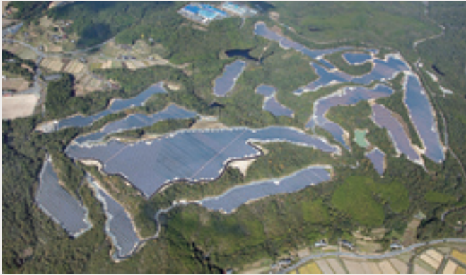
Panorama of Kumenan Mega Solar Plant
