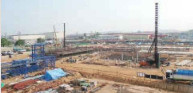
Construction on the first plant, started February 2015
