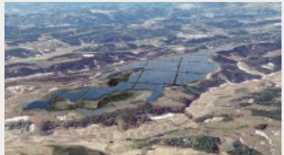
Construction site (panels are an artistic rendering)
