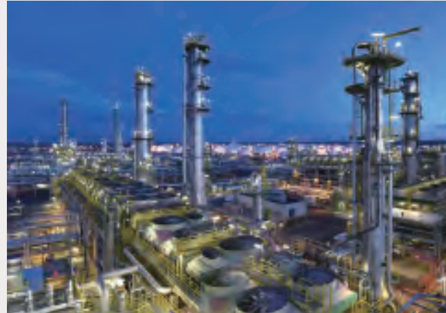
Gasoline production unit
