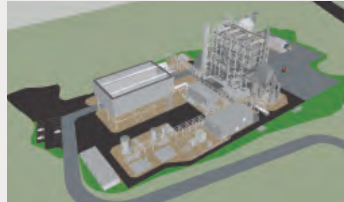
Model of completed Biomass Plant (Saga Prefecture)
