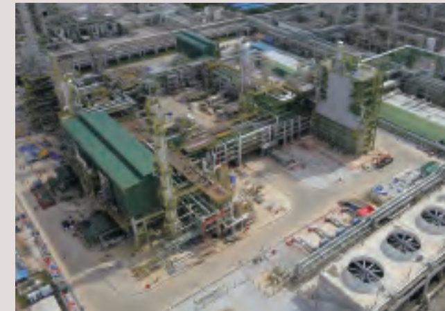
Olefin plant in operation
