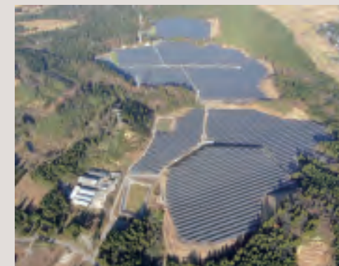
Aerial view of solar power plant
