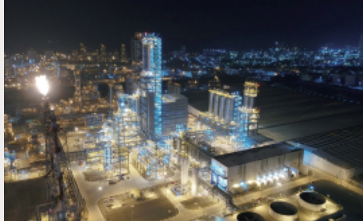
Night view of the completed polyethylene swing plant
