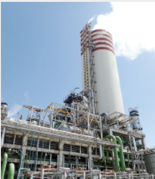
The completed fertilizer plant
