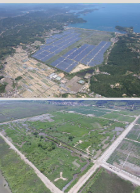
Top: Aerial view of Setouchi Kirei Mega Solar Power Plant Bottom: The Kinkai Habitat (approximately 16 hectares)
