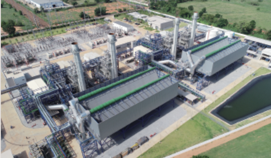
The completed cogeneration power plant
