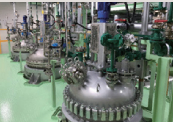
Liquid injection chambers
