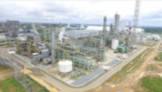
The completed fertilizer plant
