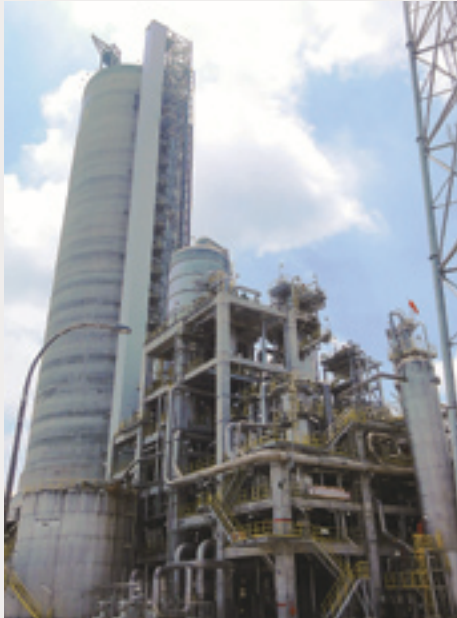
The completed fertilizer plant
