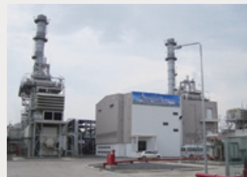
NK2 electric power plant
