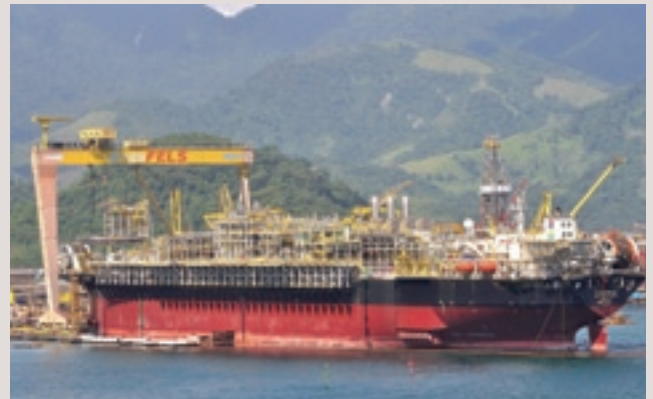
Integration of topside units at shipyard
