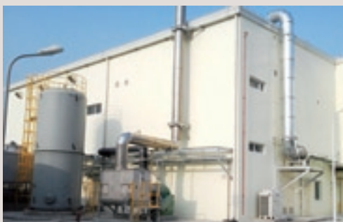
Plant in China completed December 2012
