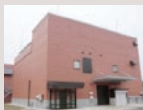
IND active ingredient facility
