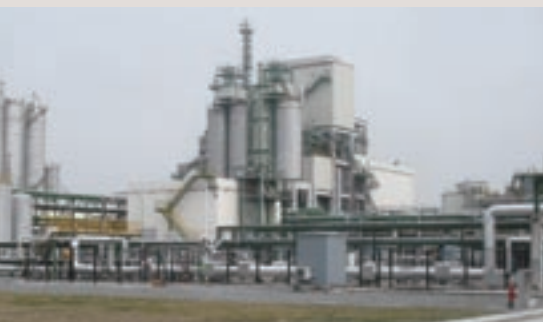
Overview of completed plant
