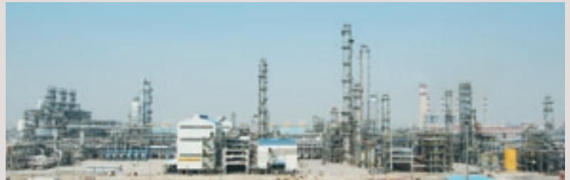
Completed ethylene plant
