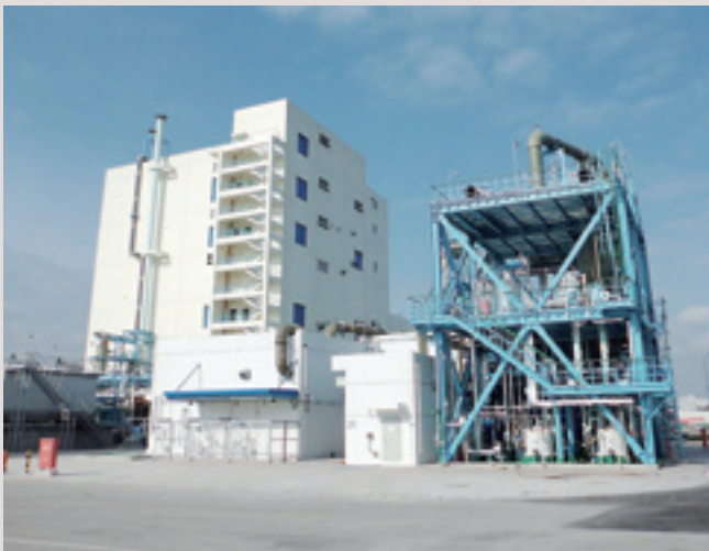
Completed plant for Chinese subsidiary of Daikin Industries
