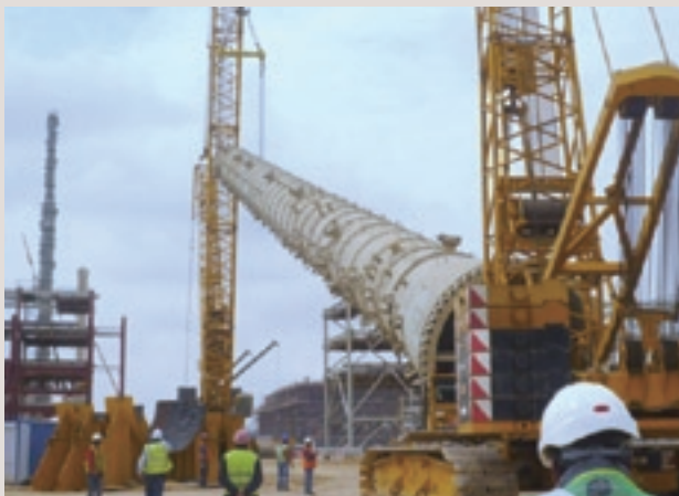
Installation of the ethylene fractionator
