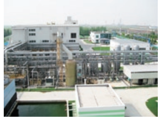
Phenolic resin plant of Sumitomo Bakelite (Nantong) Co., Ltd.
