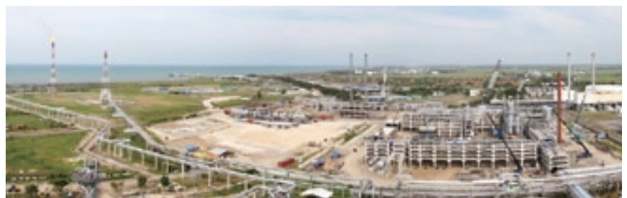
Balongan Refinery construction site
