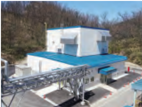
Client: Yonezawa Hamari Chemicals, Ltd. Type: High Potency API Multi-Purpose Plant Location: Yamagata, Japan
