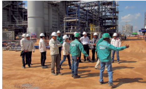
Site inspection by managers (Thailand)
