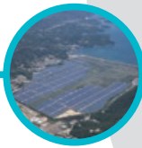
Japan Photovoltaic Power Plant
