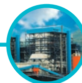
Indonesia Coal-fired power plant
