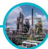
Germany Residue Upgrading
