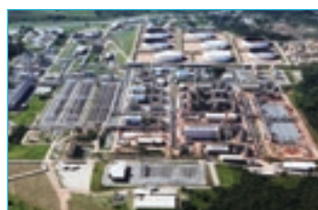
TSE gas project construction site
