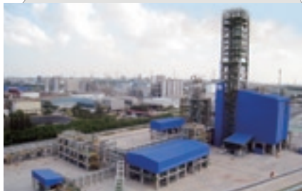
Completed LLDPE plant (Thailand)
