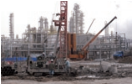
IPS-II project construction site (China)
