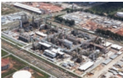
REVAP Refinery (Brazil)
