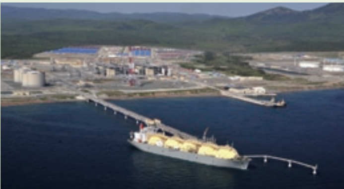
LNG plant and oil export terminal for Sakhalin Energy Investment Co., Ltd., in Russia
