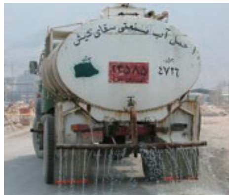
Water-sprinkling for dust prevention
