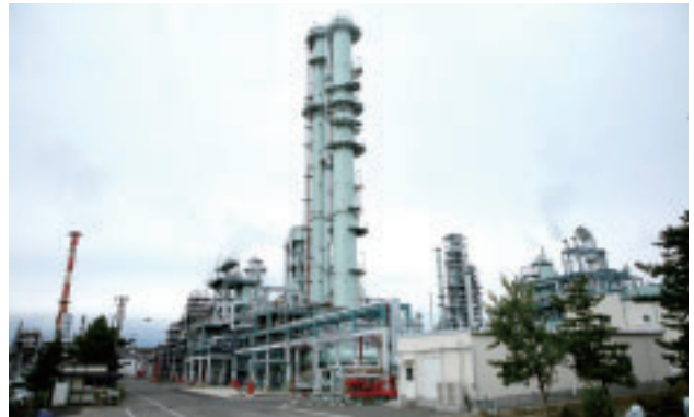
Propylene Splitter of Nippon Petroleum Refining Co., Ltd.
