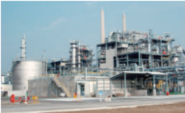
Aniline Plant II of Tosoh Corporation
