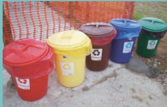
Separate collection of waste at a construction site
