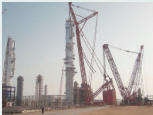
Installation of the EO / EG washtower for SABIC
