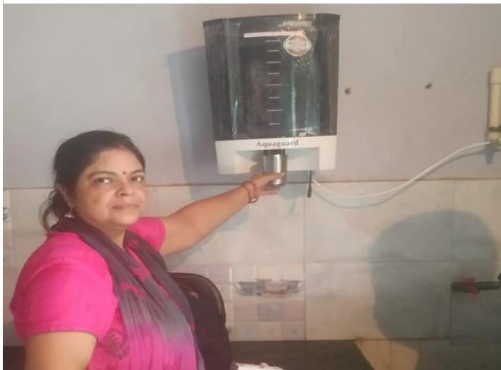
Installation of RO unit with water coolers in 10 schools in Kota district, Rajasthan
