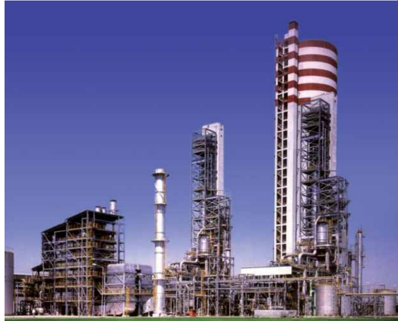
Ammonia- Urea Plant, Gadepan, - Client : CFCL
