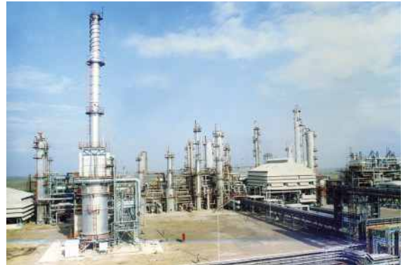
MEG Plant, Kashipur - Client : India Glycols Ltd.
