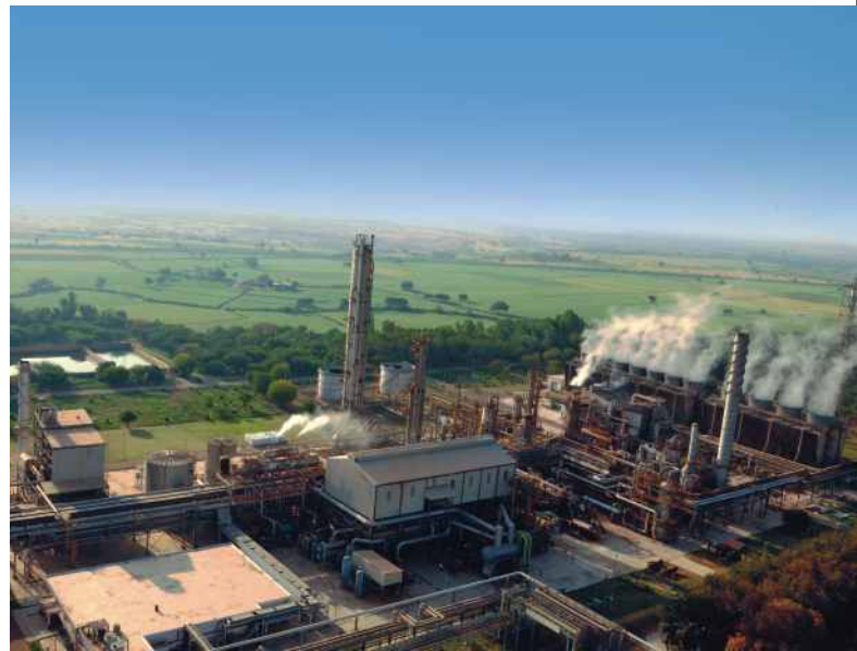
Offsites & Utilities for Ammonia - Urea Plant, Gadepan - Client : CFCL
